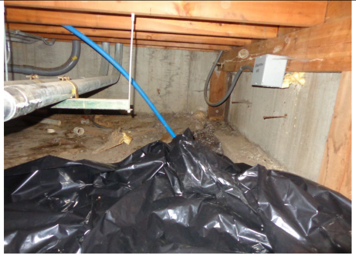
Photograph #2 – View of unattached plastic sheeting and organic materials in the crawl space.
