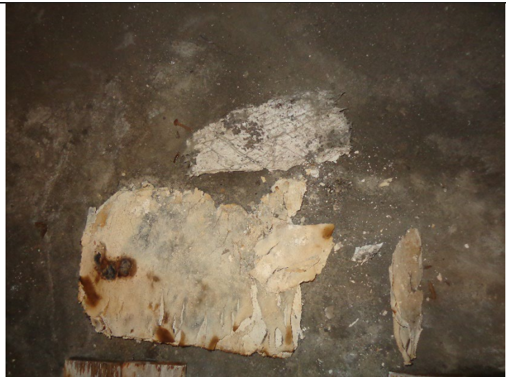
Photograph #4 – View of gypsum board debris containing mold growth in the basement's northwest corner.
